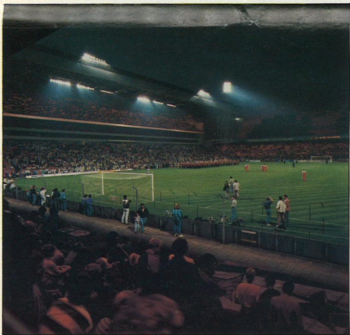
High mast lighting, supplemented by grandstand lighting at PSV Eindhoven's ground, uses the Philips Arenavision system.
