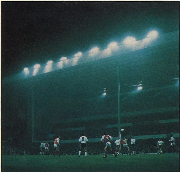
Grandstand mounted lighting, parallel to the direction of play at Tottenham Hotspur's White Hart Lane ground, lighting is by Thorn.
