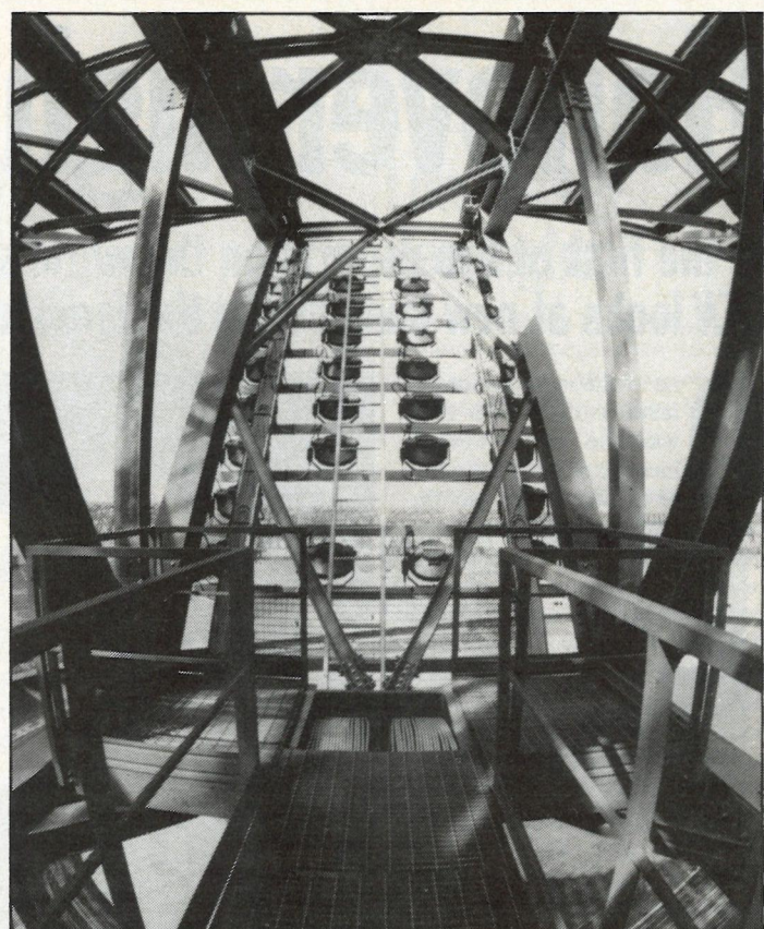
Lighting installed in the newly roofed Sao Paulo Stadium at Naples.
